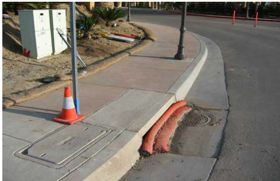
Inlet protection that blocks flow, preventing non-storm water discharges from entering drain.
