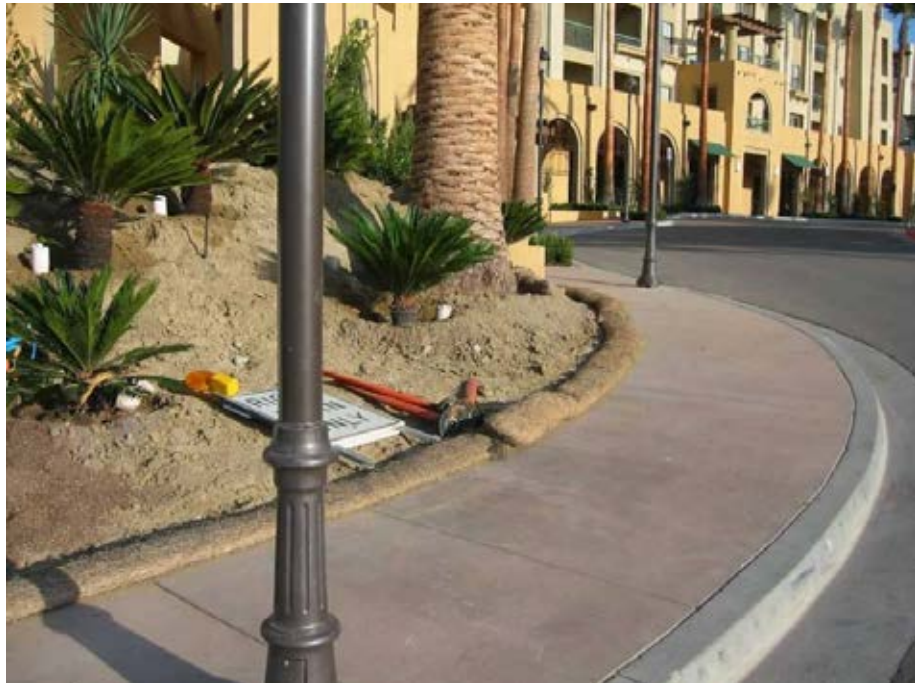
Fiber rolls as perimeter control.
