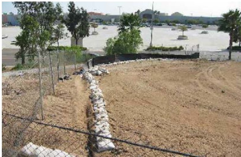
Gravel bags used as perimeter control.
