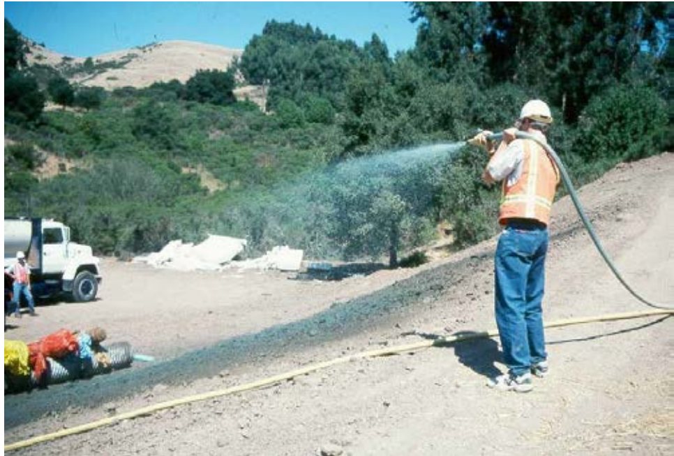
Applying hydroseed.
