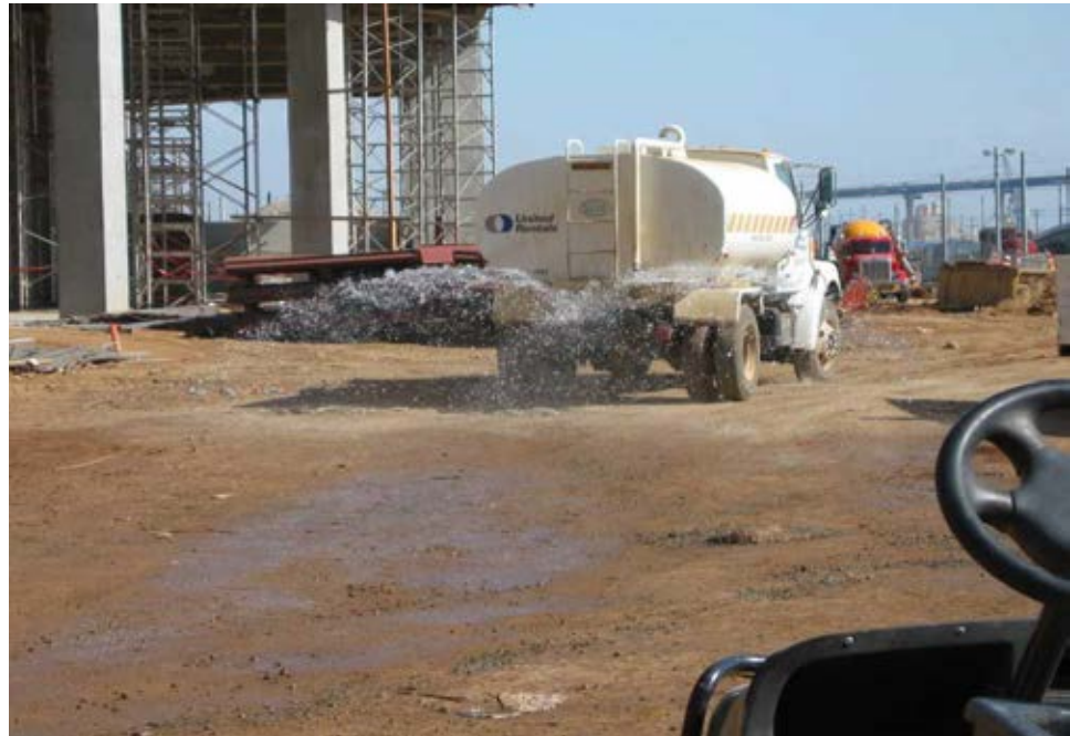
Water being applied for dust control.
